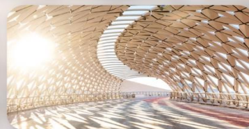
Atyrau Bridge Astana
