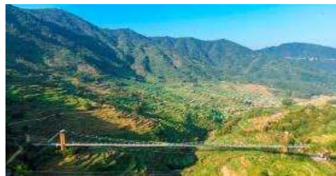
Wuyuan Glass Bridge
