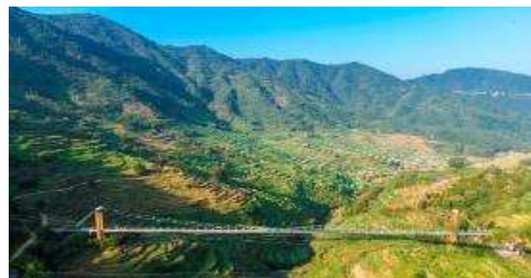
Wuyuan Glass Bridge
