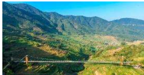
Wuyuan Glass Bridge
