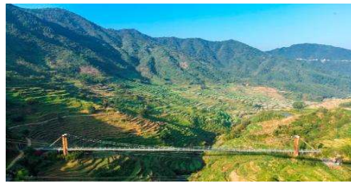
Wuyuan Glass Bridge
